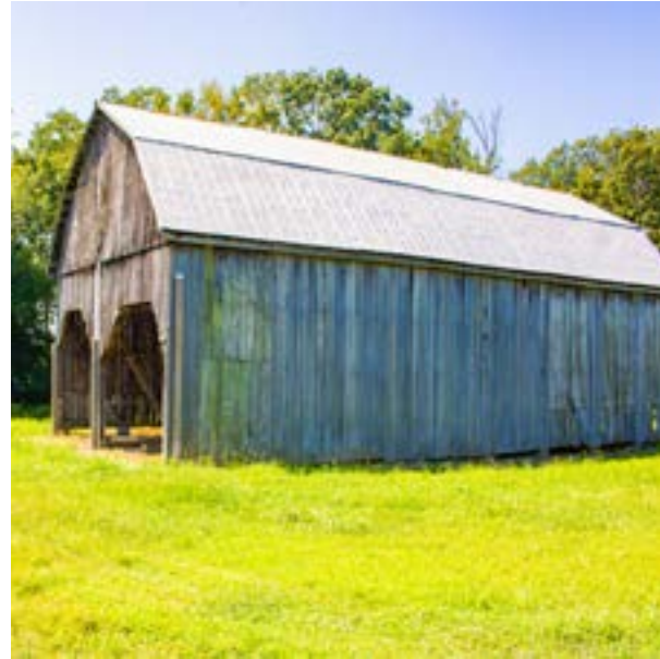
Figure 2.09: Existing Barn, Focus Area 2. Credit: Joe Ignatius
