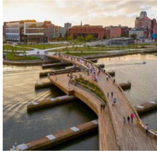
Figure 3.16 Providence Pedestrian Bridge Credit: Steve Kroosma
