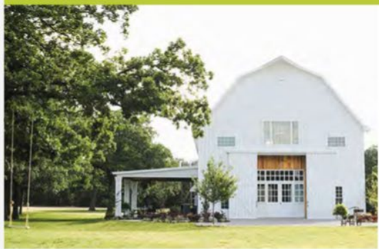
RENOVATED BARN + EDUCATION CENTER
